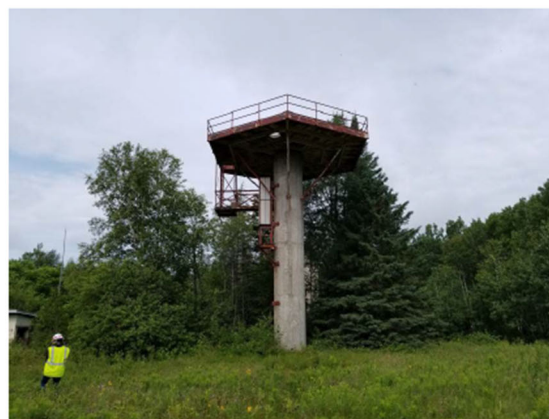
Radar towers. Three of four top platforms have been dismantled as of 2013 (2017).
