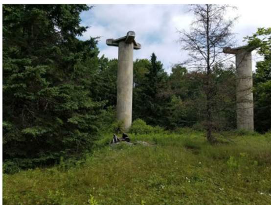
Radar towers. Three of four top platforms have been dismantled as of 2013 (2017).
